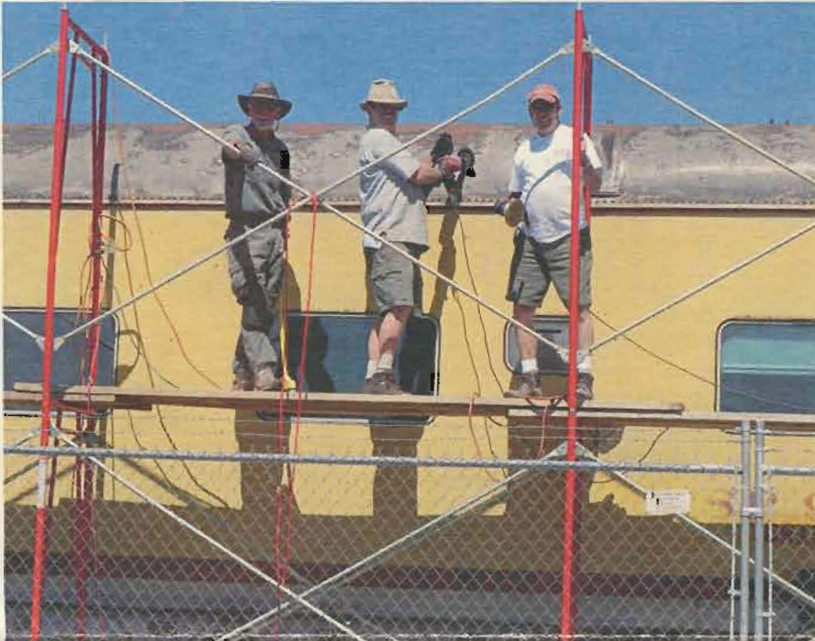
Bob Williams, Steve Disbrow and Don Clukey; three local day laborers, grind away on rusty sleeper roof.
